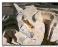
The sockets for a removed iron clamp.
