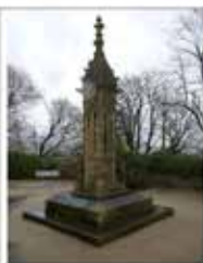
B: General view of the Pinnacle
