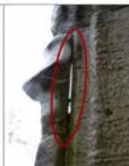
E: Open joint at junction of cill and corner pier. Joint requires cleaning out, pack pointing and finish pointing to arrest water ingress and frost damage. Horizontal crack in stone pier. Requires pinning to prevent detachment, if lower or upper blocks are loose carefully remove, back bed, pin and point to arrest water ingress and frost damage
