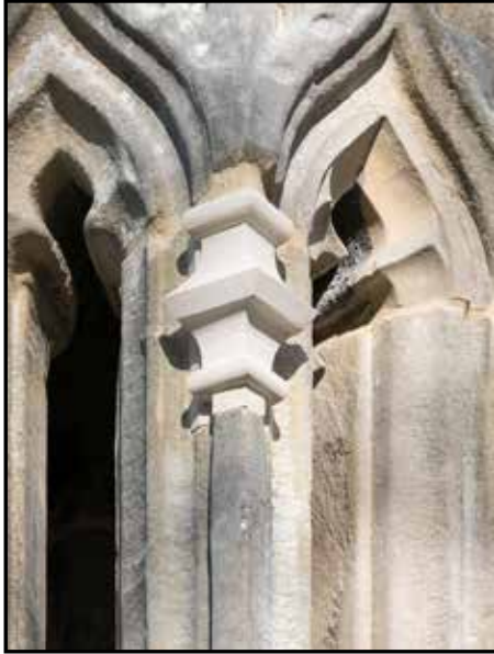
The new repairs using magnesian limestone from Jackdaw Quarry.
