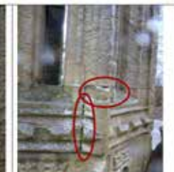
E: Open joint at junction of cill and corner pier. Joint requires cleaning out, pack pointing and finish pointing to arrest water ingress and frost damage. Horizontal crack in stone pier. Requires pinning to prevent detachment, if lower or upper blocks are loose carefully remove, back bed, pin and point to arrest water ingress and frost damage
